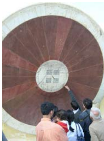
The Equinoctial Instrument is a vertical hole in the wall of one of the instruments. The lower surface is inclined at the latitude of Delhi (28 degrees 39 seconds) so that when the Sun enters into the chamber and falls on a peg only when it is in the equinoctial position (exactly above the equator), twice a year.
