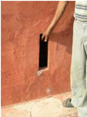
The Equinoctial Instrument is a vertical hole in the wall of one of the instruments. The lower surface is inclined at the latitude of Delhi (28 degrees 39 seconds) so that when the Sun enters into the chamber and falls on a peg only when it is in the equinoctial position (exactly above the equator), twice a year.
