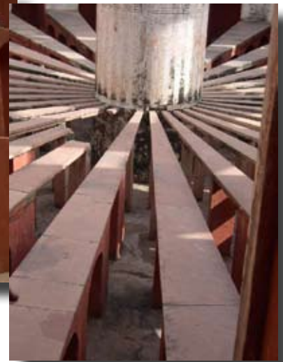
The Ram Yantra is a multifloor version of an Azimuth Instrument which also measures the altitude of heavenly bodies. At sunrise the shadow falls on the central pillar at what is essentially zero altitude.
